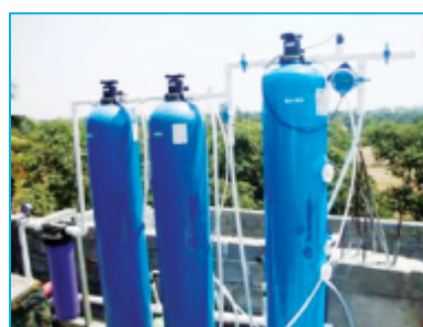
D.M. Water Plant (With & Without Mix Bed)
